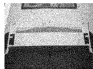
Center horizontal structural component is isolated consequently the fabric does not engage the center structural component.
