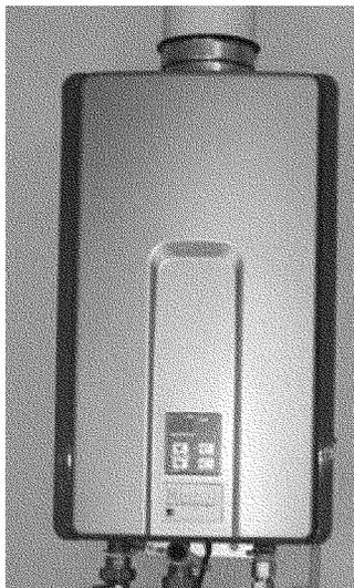
Figure 6. Japanese tankless gas water heater
